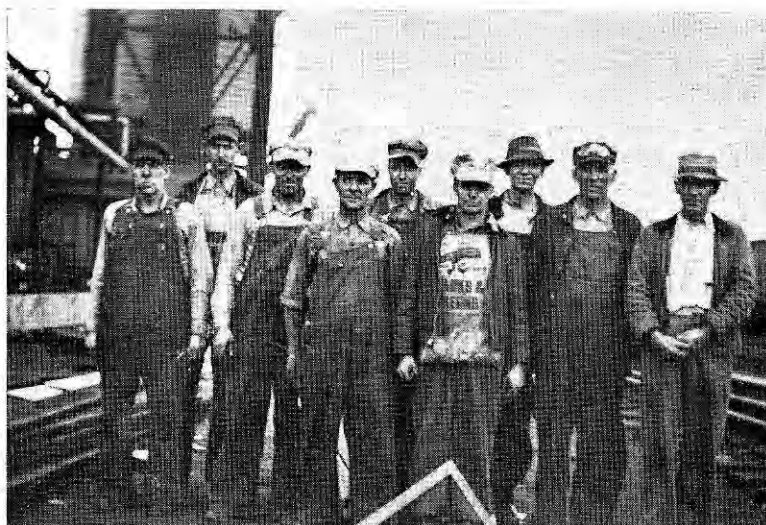
Repairing Office Building, Albion Terminal. From left to right, G. M. Holder, Glen Patton, G. W. Graft, Jr., G. T. Wilson, H. J. Callahan, A. E. Soltis, H. E. Reagle, William Wallace, and A. J. Redfoot, Foreman.
